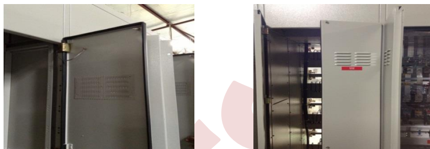
Figure 8 : Inspections of overall dimension of switchboard, check overall paint work, door locking device, door gasket, door hinges, door cut-out holes
