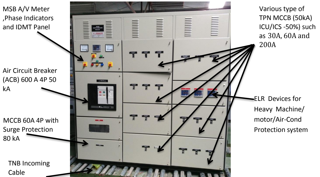
Figure 2: Compartment devices installed in MSB
