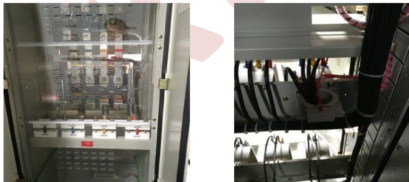
Figure 9 : Inspections location of feeder entry point, cables and earthing conductors, cable tightening, and bus bars clearance
