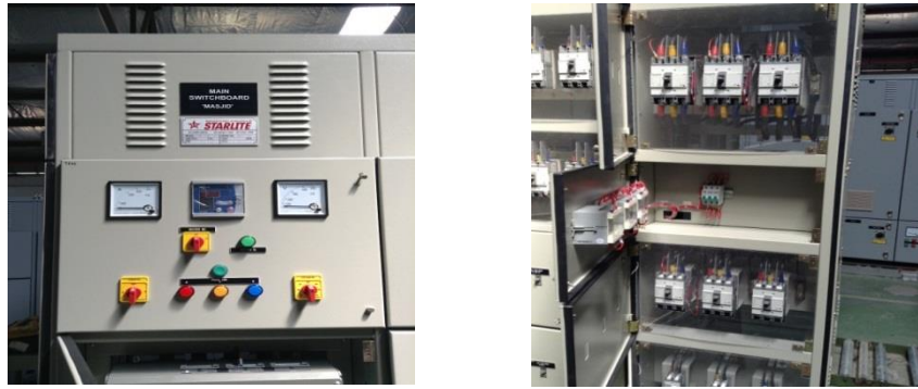
Figure 7 : Inspections of fitted components check and verify the brand, model, and identification components installed (breakers, current transformers (CT), fuses, ammeters, voltmeters, power meters and protection relays etc.)
