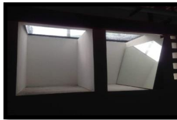
Daylighting using reflective mirror
